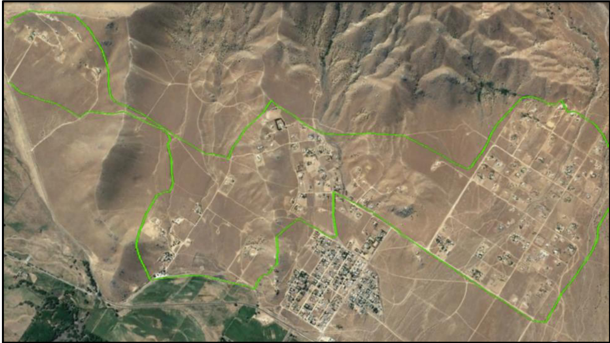
Figure D.50. Community is situated at base of slope. Adjacent community consists of dense clustering of homes — mostly trailers and mobile homes with poor separation.
