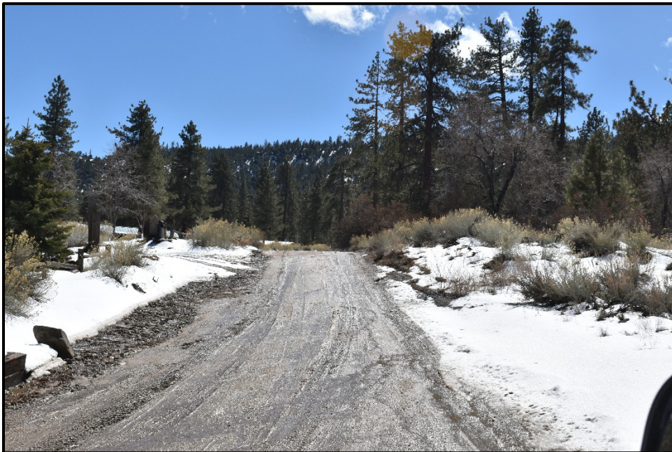
Figure A.5. Photograph showing a wet unsurfaced road.
