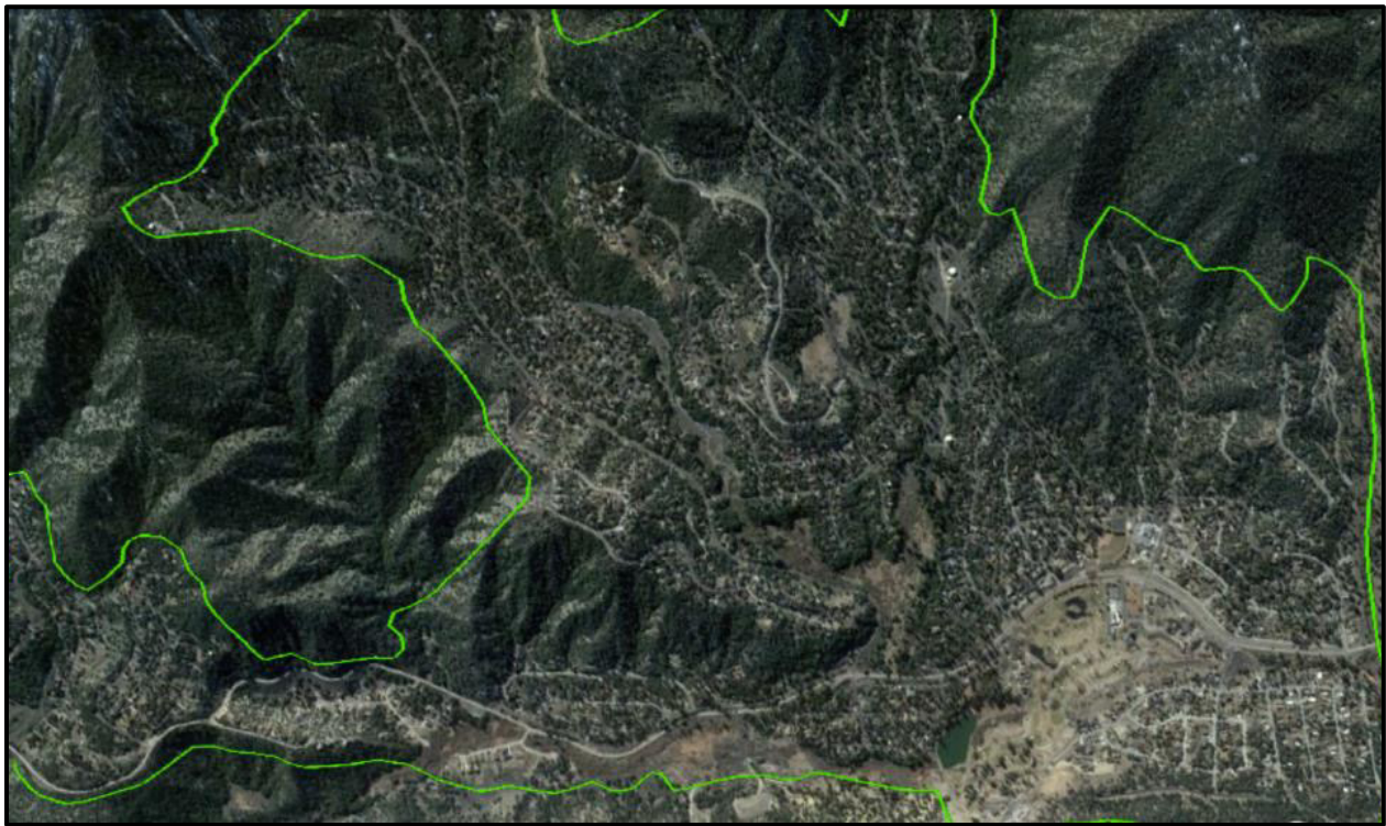
Figure D.3. All homes have wood siding, some with exposed propane tanks. Many homes are situated mid-slope with fuels below.
