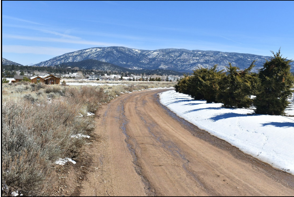
Figure 2.16. Unsurfaced road, example 2.
