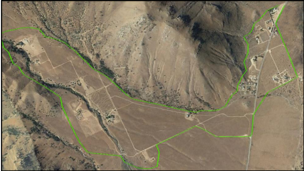
Figure D.52. Community with dispersed ranch homes in a canyon. Larger properties have good defensible space. Smaller properties have limited defensible space.
