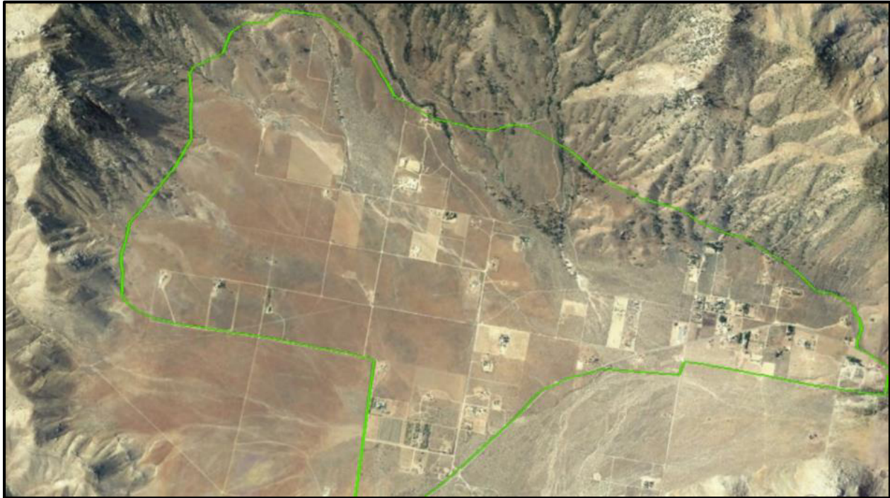
Figure D.53. Community is situated along base of slope. Vegetation consists of sage brush with grass intermixed. Homes have limited defensible space.
