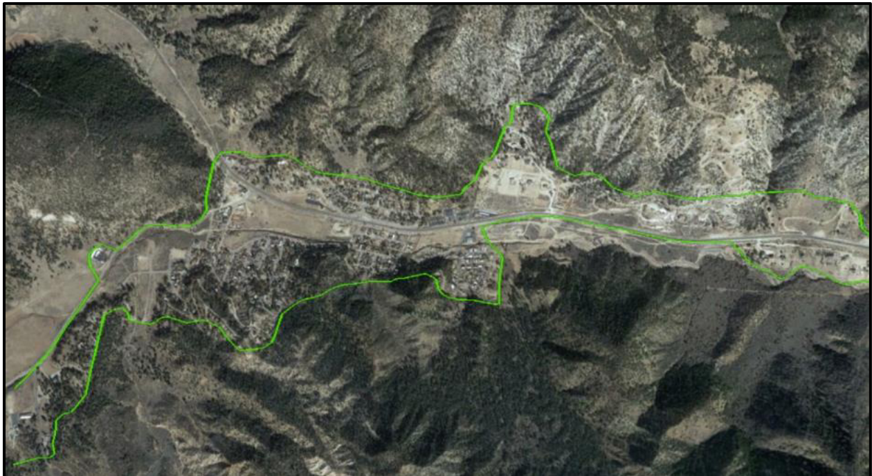
Figure D.6. Majority of homes have limited defensible space. Structures have poor separation in between; high probability of structure-to-structure ignition.
