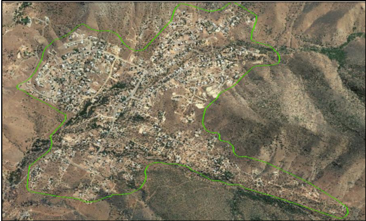
Figure D.34. Community in a canyon with multiple ridges. Heavy fuel loading noted throughout community. Most structures have heavy fuels in between.
