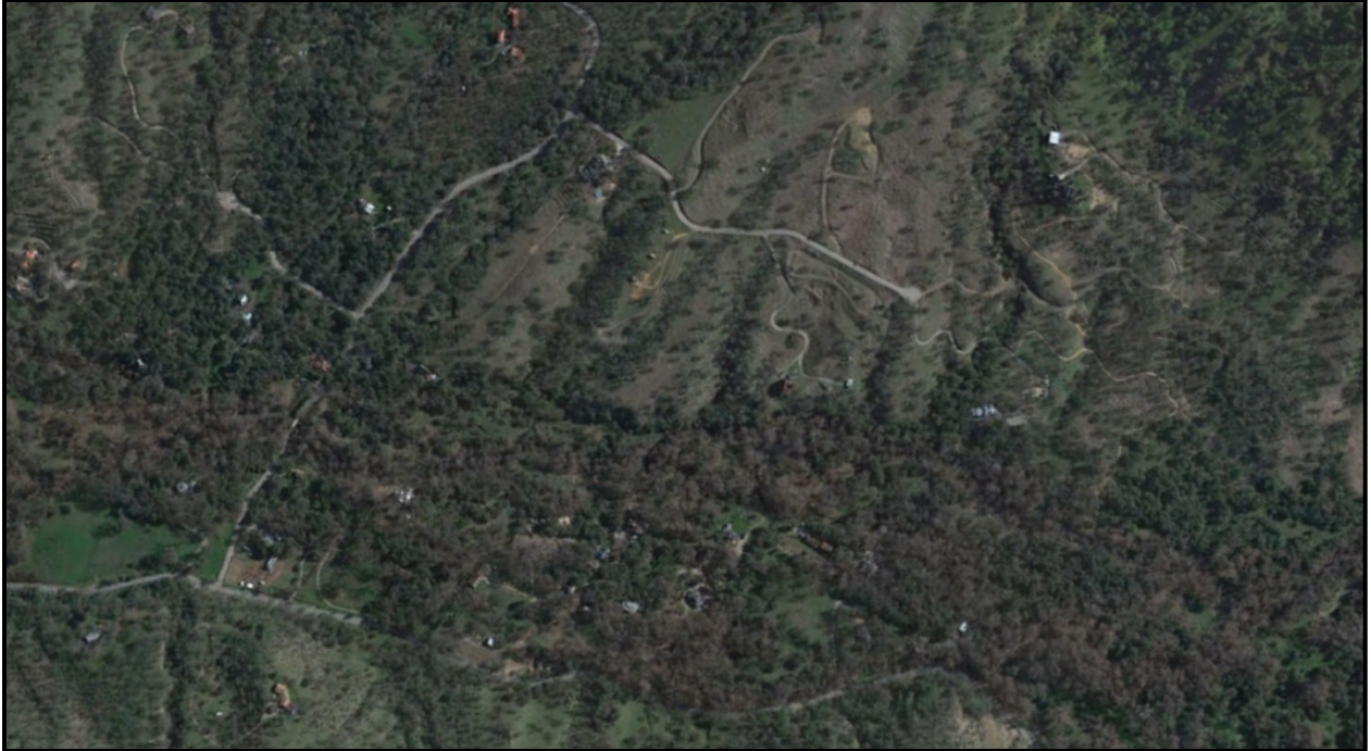
Figure D.8. Larger lot sizes with structures that are further apart and closer to more moist riparian vegetation. One road in and out of polygon. Red markings are project WUI boundaries. Source: Google.
