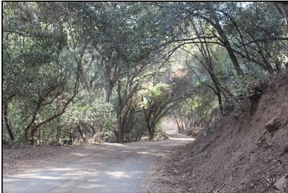
Figure 2.12. Example of unsurfaced, narrow, and winding road.
