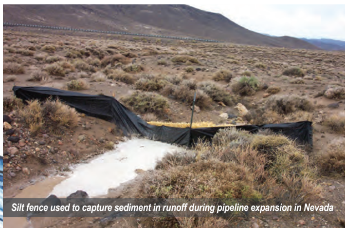
Wire-reinforced silt fence for erosion control on a construction site
