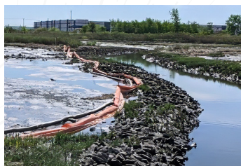
> SPILL RESPONSE AND NRDA
